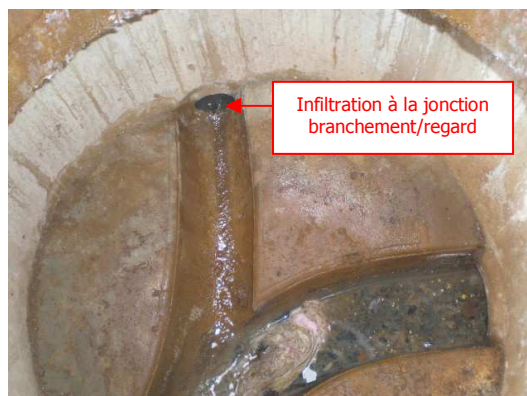
FIGURE 13 : INFILTRATION PLACE SAINT-MARTIN
